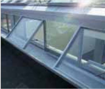
Skylight for ventilation purposes in Aabenraa Hospital (Denmark)
