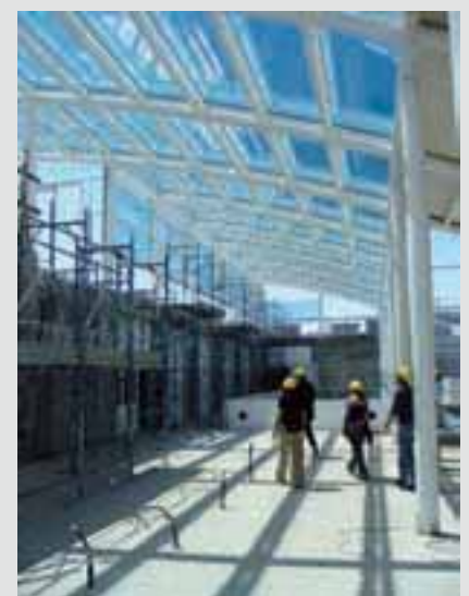
Glazed buffer space at Meyer Children's Hospital (Italy)
