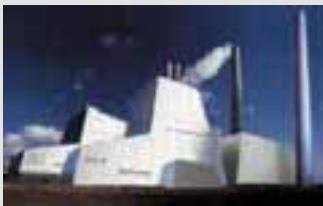
The CHP plant Avedøre 2 in Denmark
