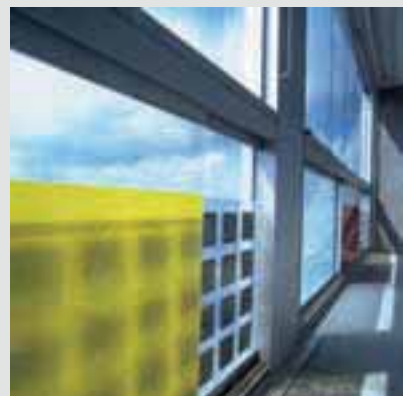
Multi-functional PV system from Kollektivhuset in Copenhagen (Denmark)
