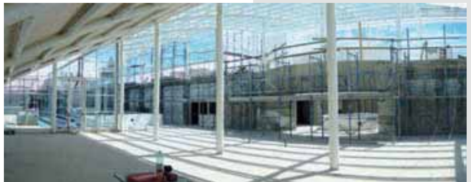
Glazed buffer space at Meyer Children's Hospital (Italy)
